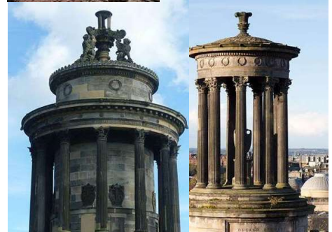
● Robert Burns Monument, Calton Hill, Edinburgh, Scotland Dugald Stewart Monument, Edinburgh, Scotland
